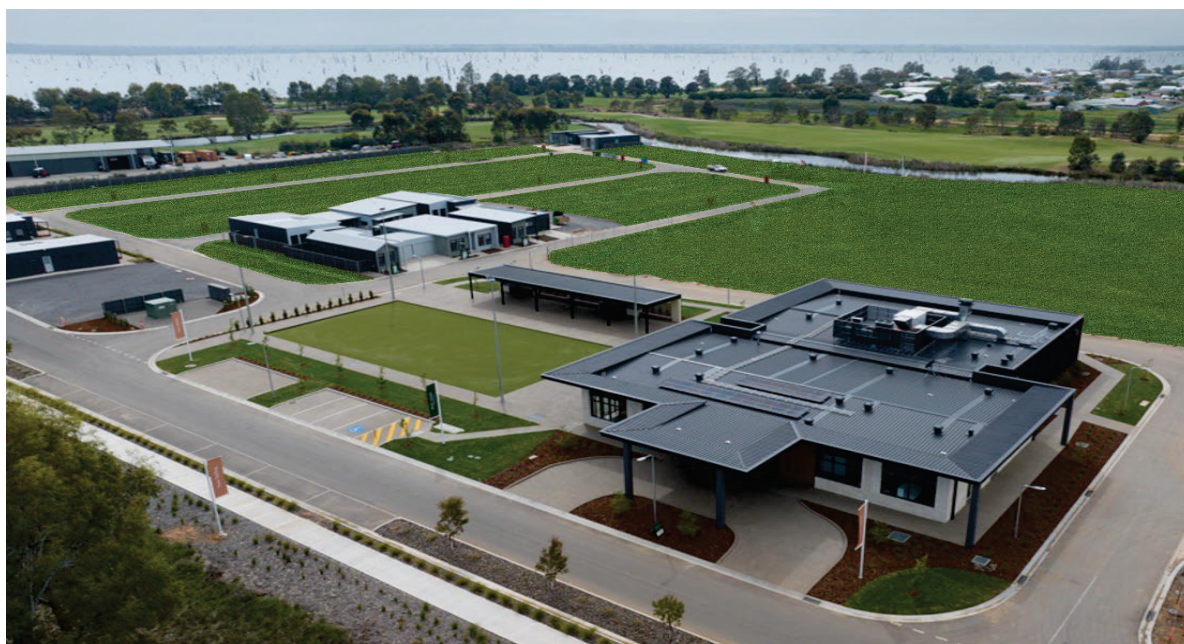
Zest Living Yarrowonga – site view with Clubhouse in foreground and 6 completed homes in the middle ground
