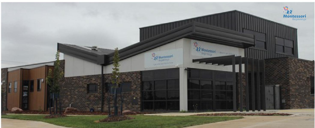
Outside view of the Greenvale centre
