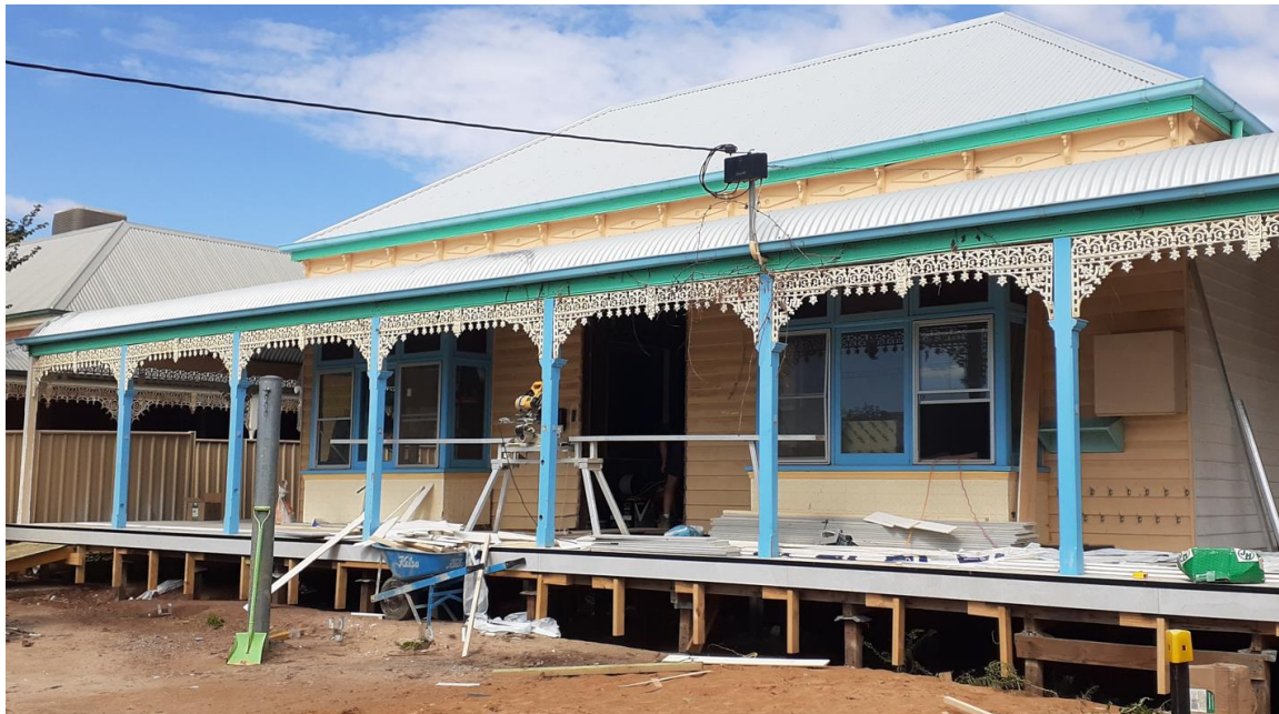
Long day care centre expansion site: Swan Hill at Mar-22
