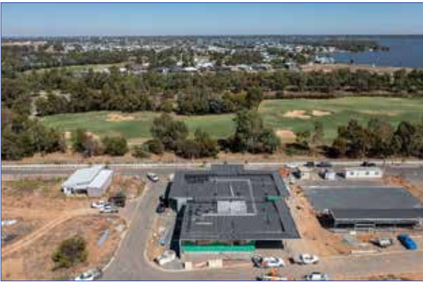
Community Centre under construction
