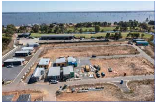
Display village and first homes under construction
