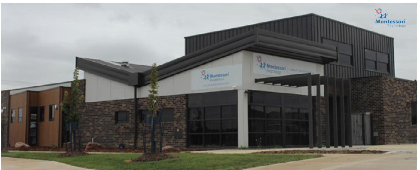
Outside view of the Greenvale centre
