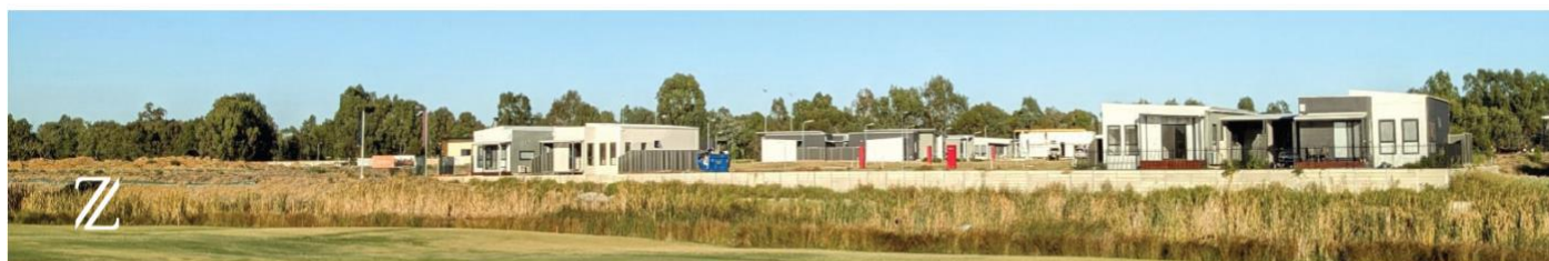
View of completed houses at Zest Living, Yarrowonga
